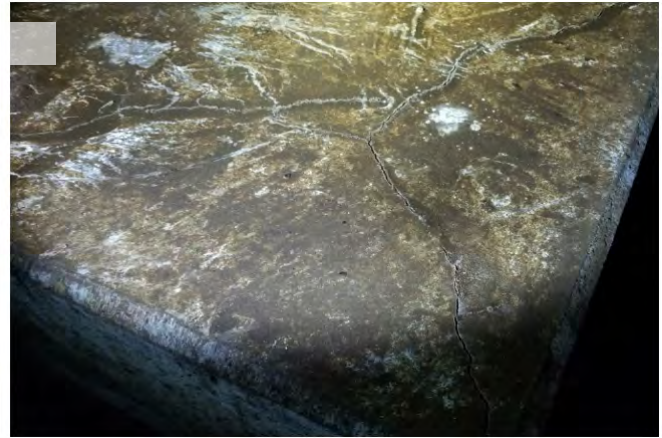
Figure 4: ASR footing cracks in Equestrian Trails Tank
