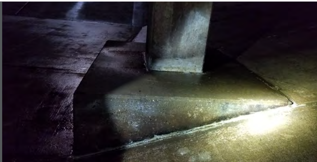
Figure 5: Typical partially embedded column footing at Equestrian Trails Tank
