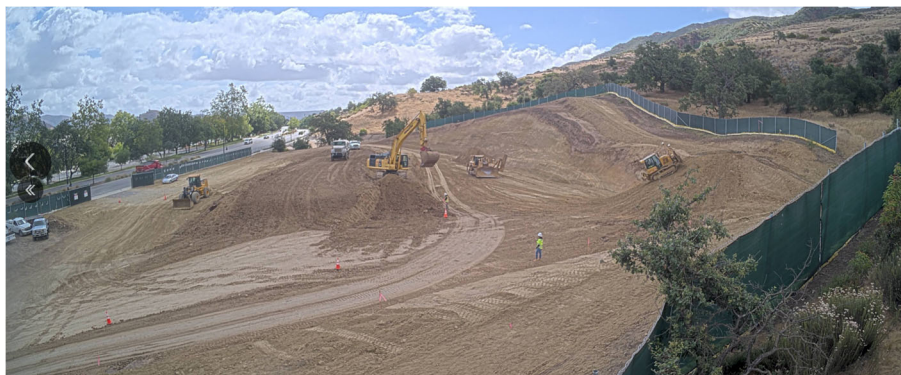
Mass Grading of AWPF site
