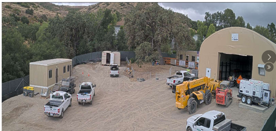
AWPF Owner's Trailer, Walsh Trailer, and Warehouse
