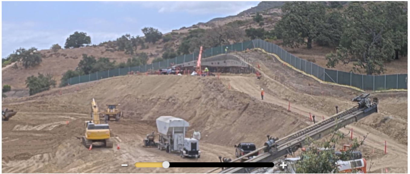
Soil Nail Wall Construction
