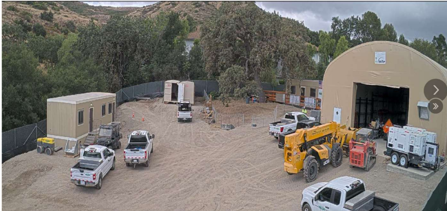
AWPF Owner's Trailer, Walsh Trailer, and Warehouse
