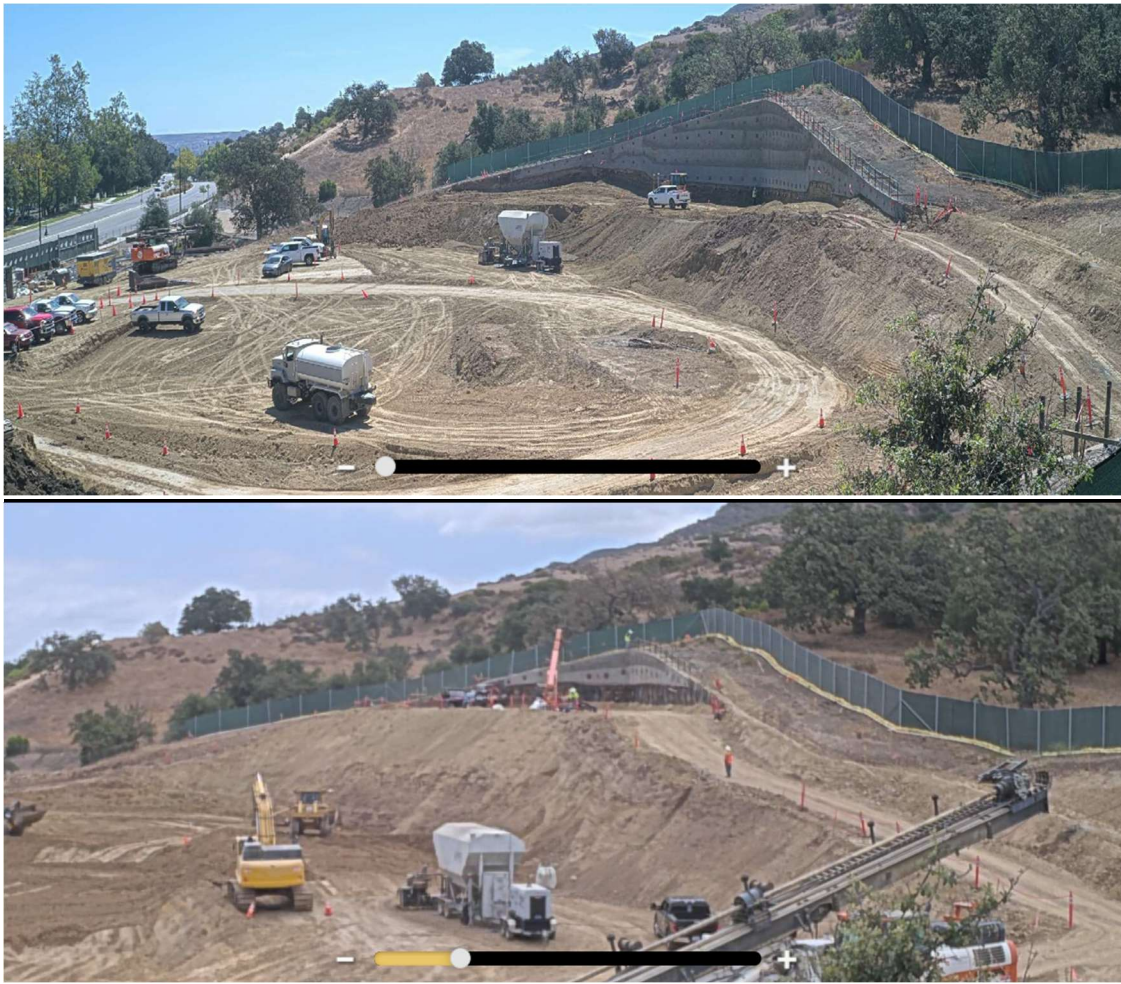
Soil Nail Wall Construction
