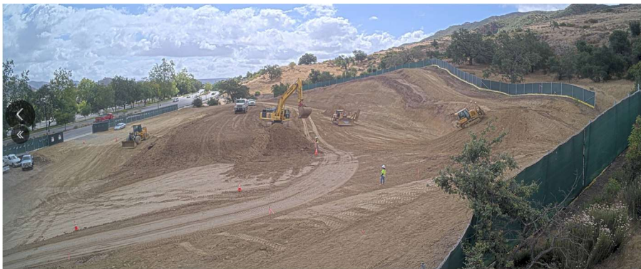
Mass Grading of AWPF site
