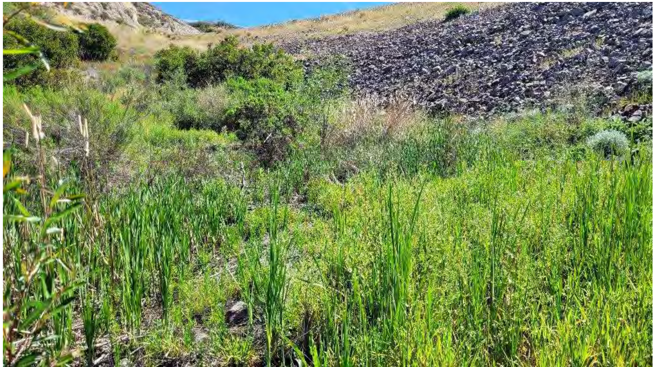
Photo 3: View of downstream toe of the right side of the main dam looking toward the downstream slope.
