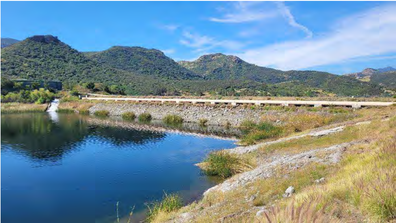
Photo 4: View of the aquatic vegetation along the upstream slope of the saddle dam.
