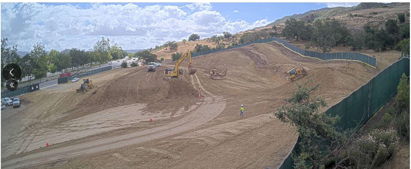
Mass Grading of AWPF site
