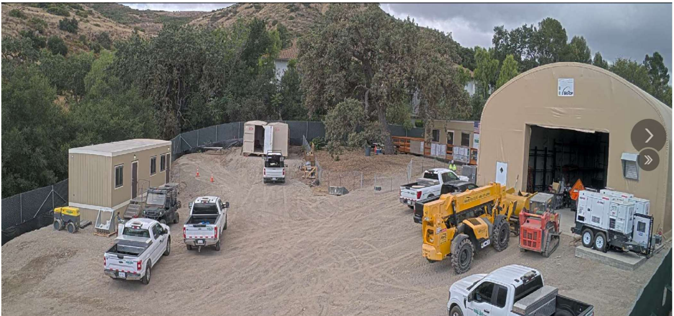
AWPF Owner's Trailer, Walsh Trailer, and Warehouse
