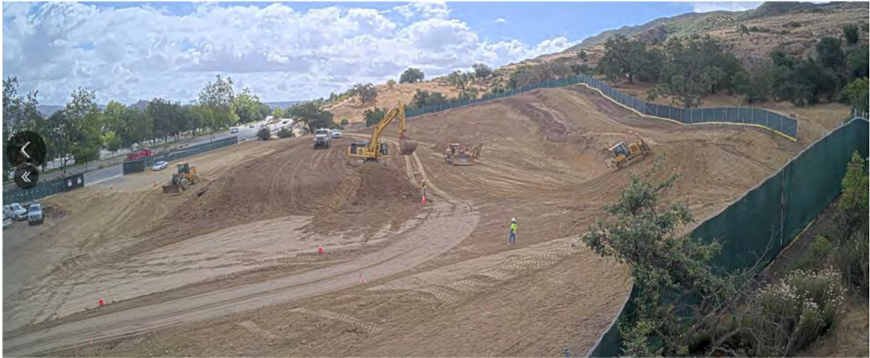
Mass Grading of AWP site
