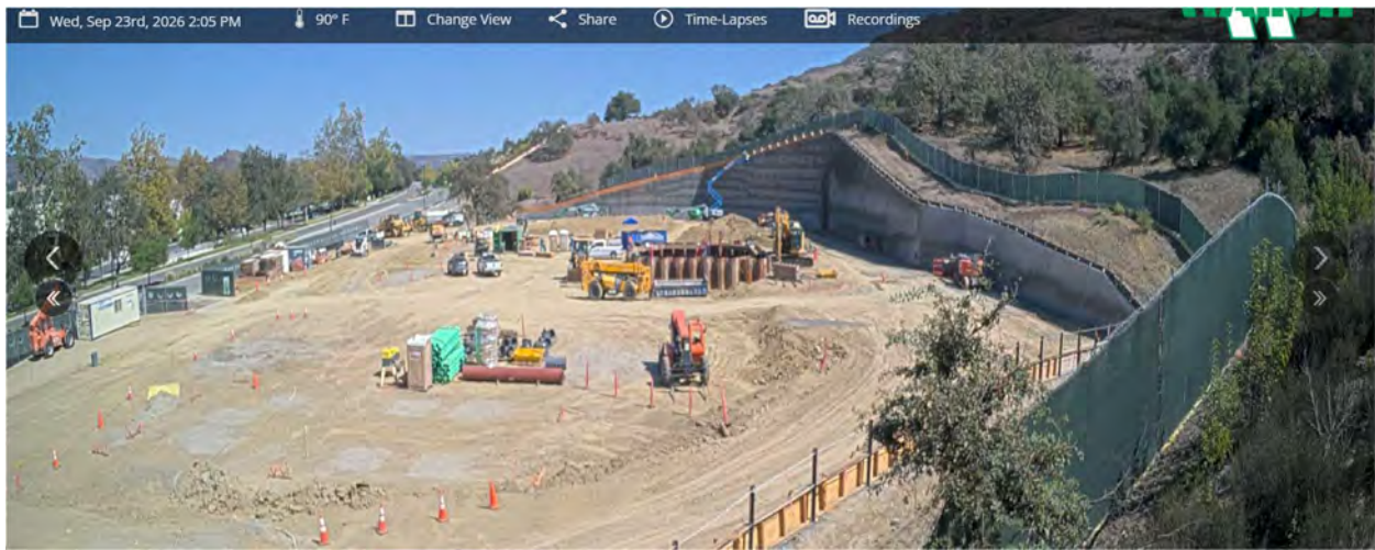
Completed soil nail wall, Waste EQ tank construction
