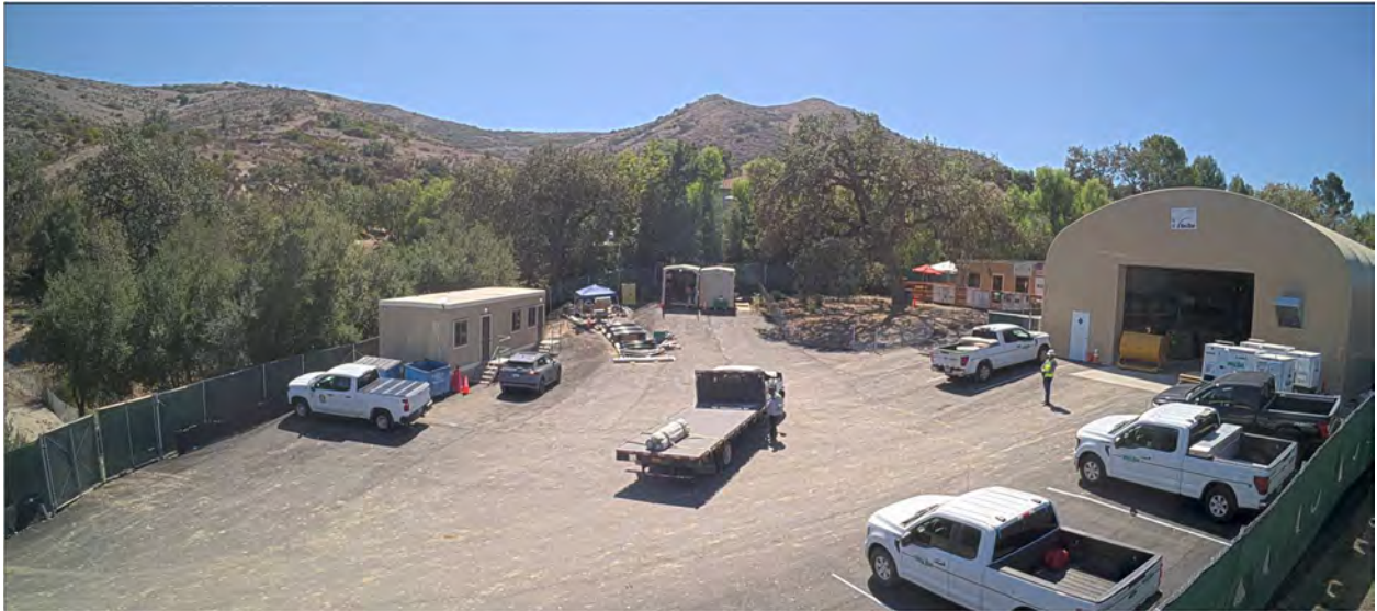
Laydown yard with temporary paving
