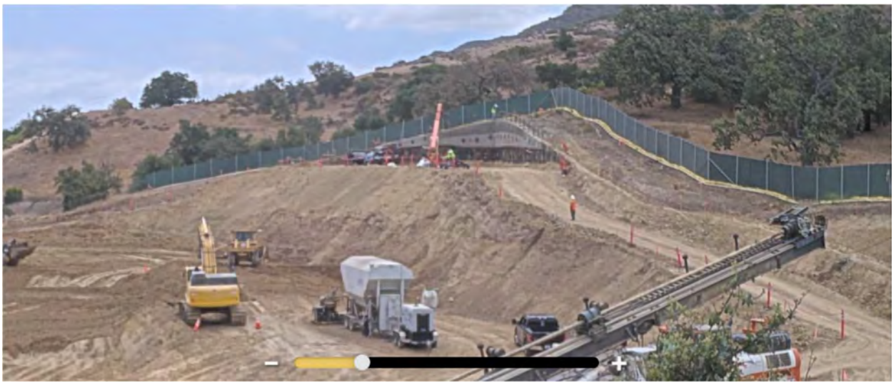
Soil Nail Wall Early Construction
